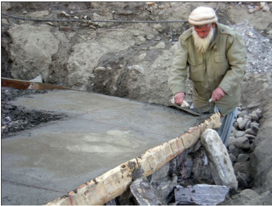
210 feet foot bridge being built, Gilgit Baltistan
