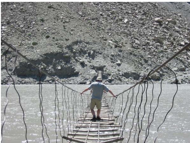
Example of a foot bridge crossing the Indus River prior to the devastating floods, Gilgit Baltistan
